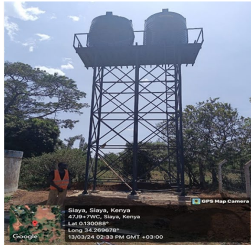
The completed 9m high tower carrying two 10,000 litre water tanks.
