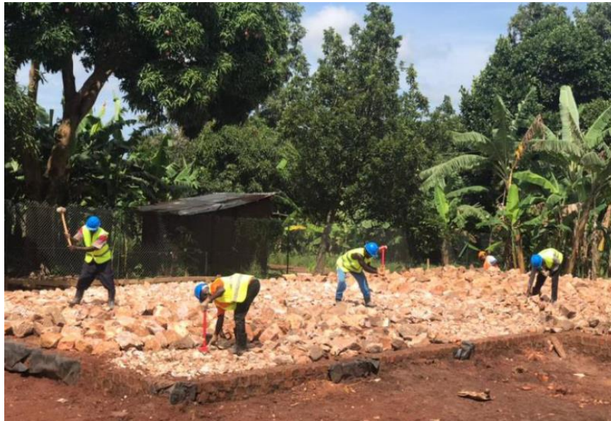
3-Classroom Block during construction (November 2023)
