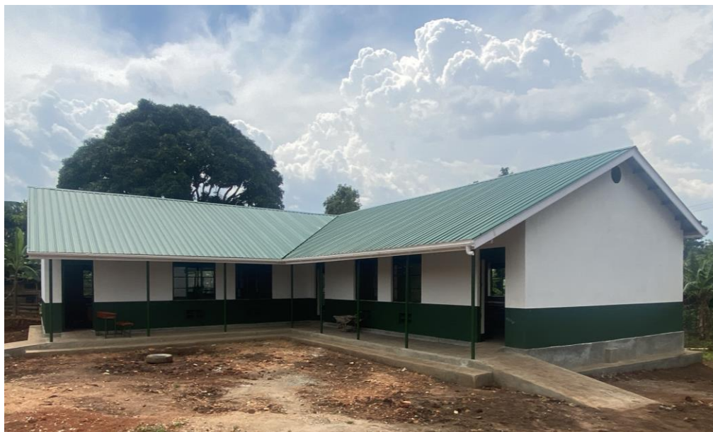
Completed 3-Classroom Block
