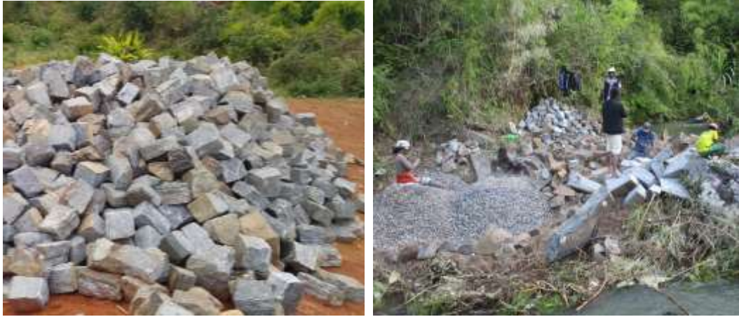
Figure 3 Building stones and gravel being prepared
