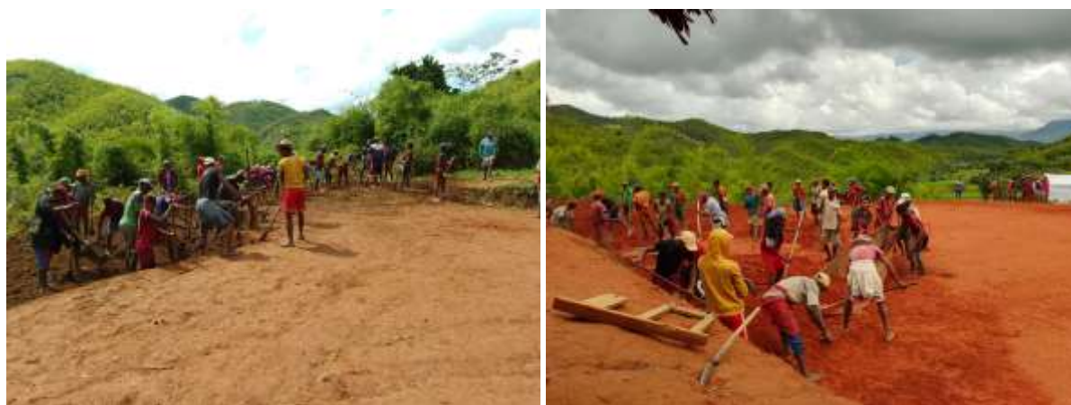
Figure 2 Earthworks (levelling of the land) by beneficiaries
