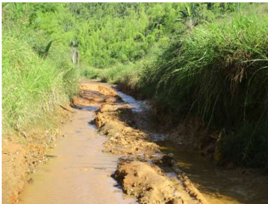
Figure 7 Condition of the road to Tsaratanana
