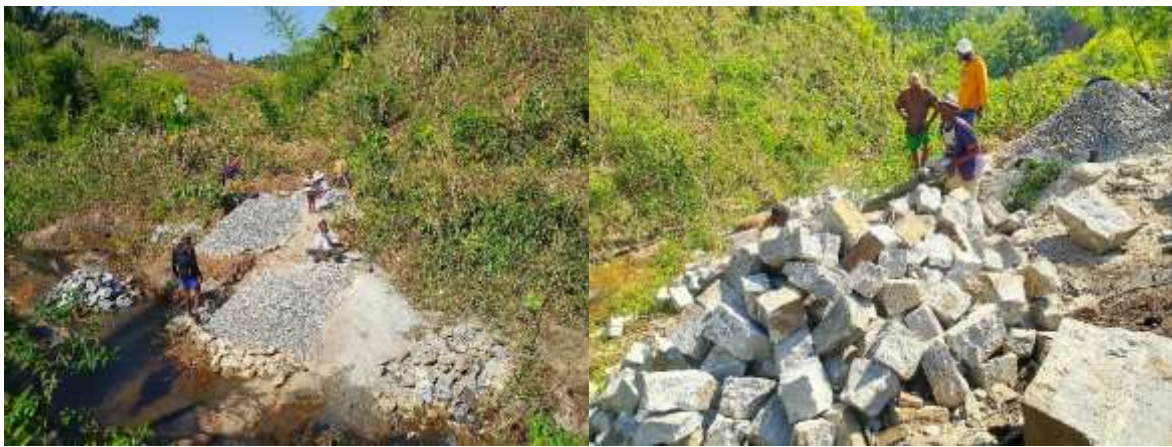
Figure 5 Stone & gravel crushing phase
