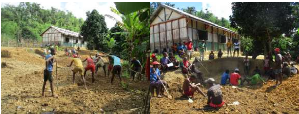
Figure 2 Beneficiaries level the land for construction at Sandrakely Primary School
