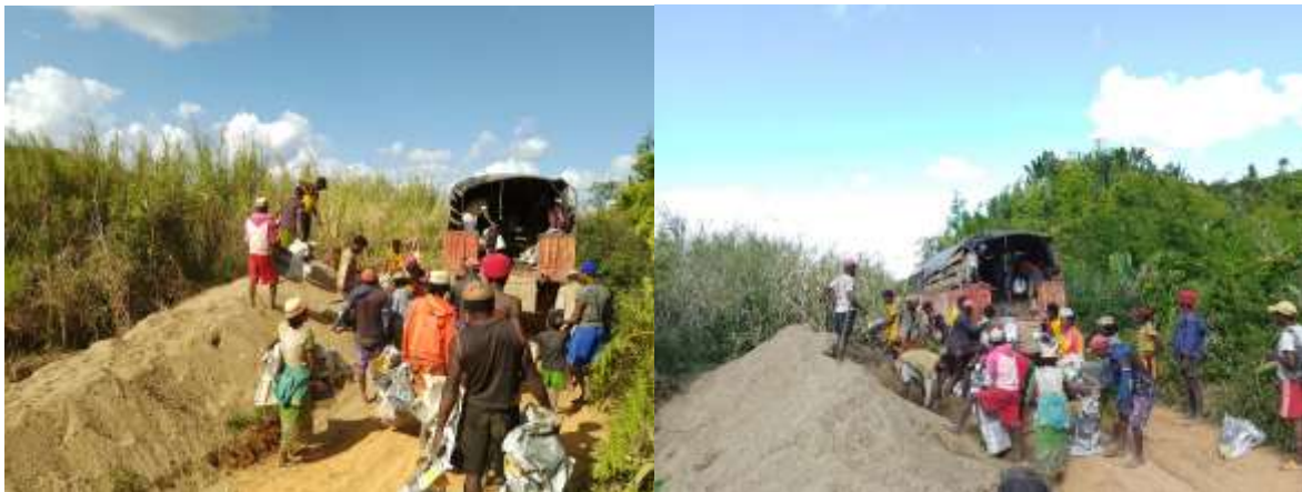
Figure 6 Sand transport by truck
