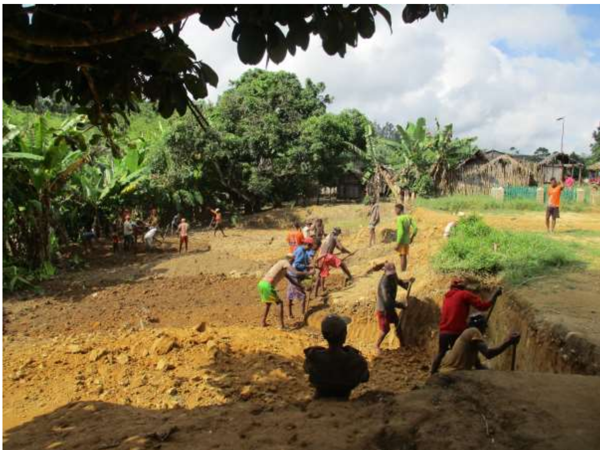
Figure 1 Earthworks at the site to flatten land in preparation of building.
