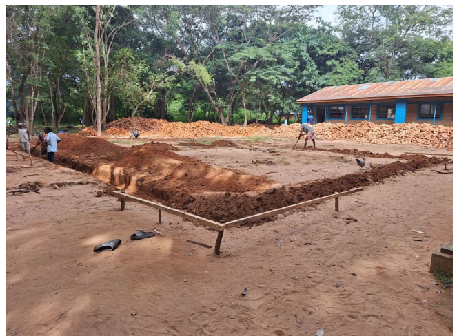
Foundations were dug in May 2024
