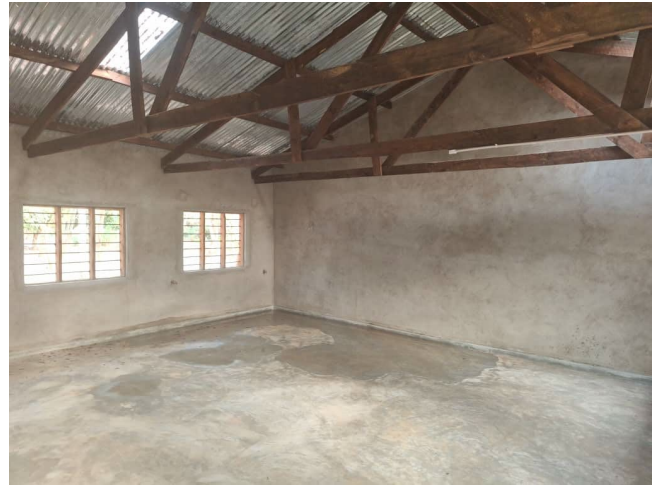
September 2024 – plastering and flooring completed
