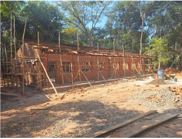
Building progress August 2024
