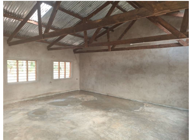
September 2024 – plastering and flooring completed
