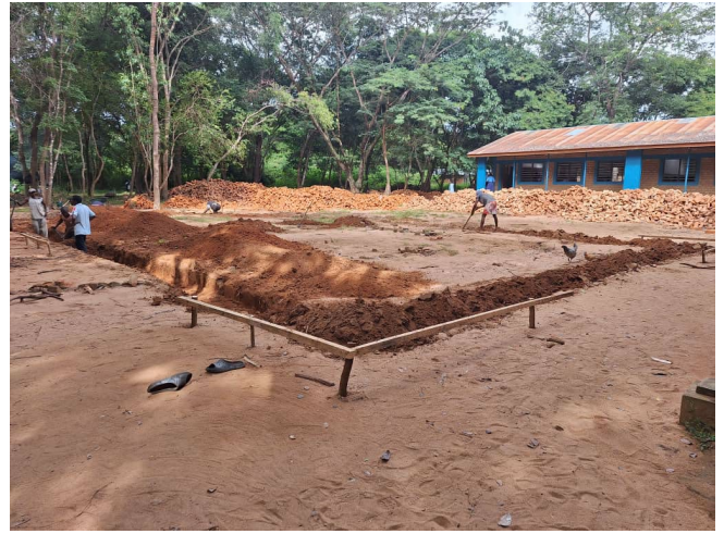
Foundations were dug in May 2024
