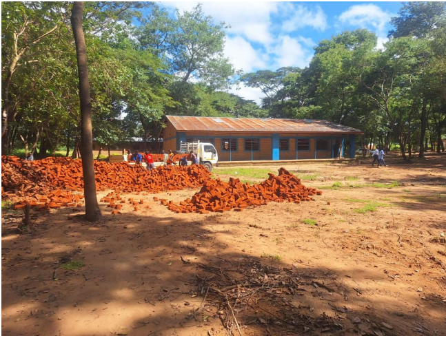
Bricks were transported to the school site in April 2024
