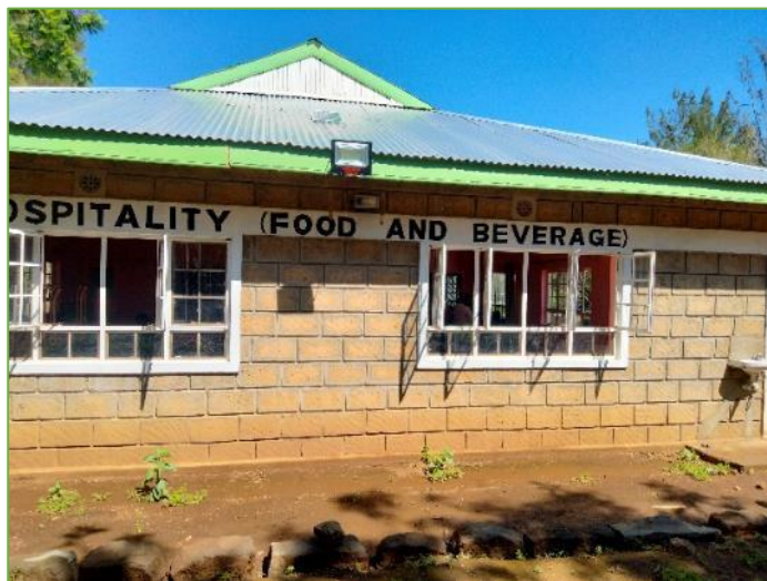
Food and Beverage centre security lighting
