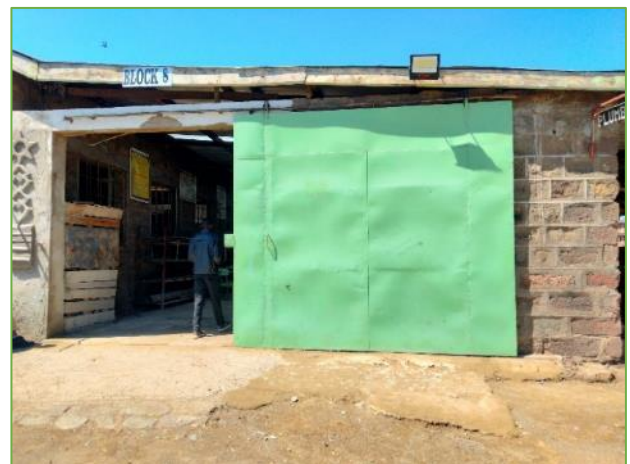
Plumbing and Masonry lecture hall
