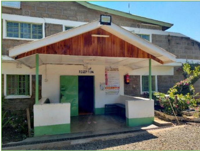
NTTI Front office security lighting
