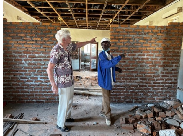
Architect Jan discussing wall division to antenatal ward.
