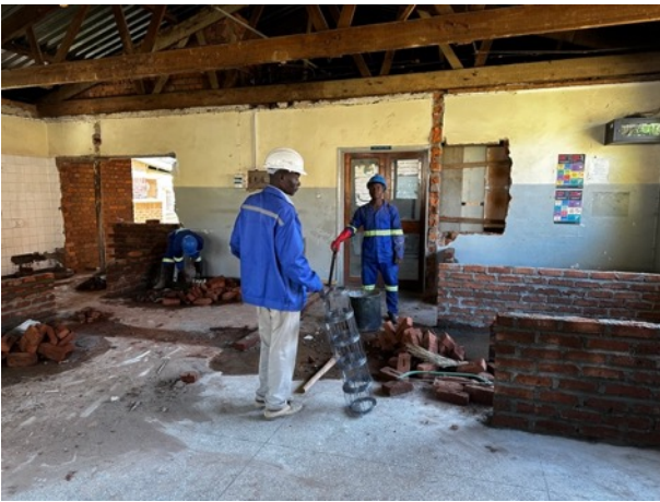
Delivery Room internal walls being built.
