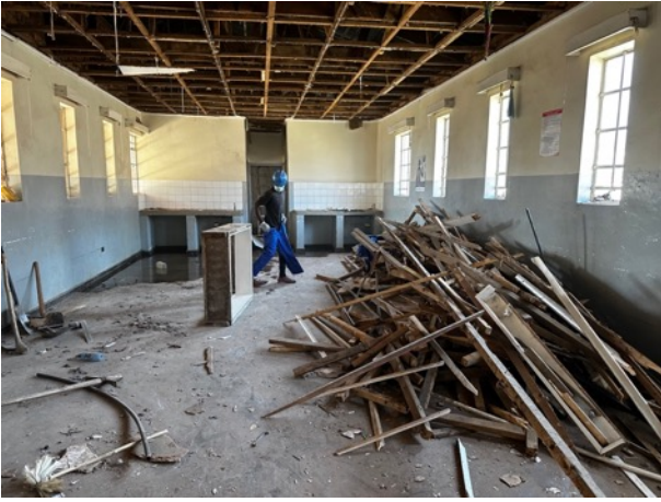
Removal of rotten timbers and old ceiling in postnatal ward
