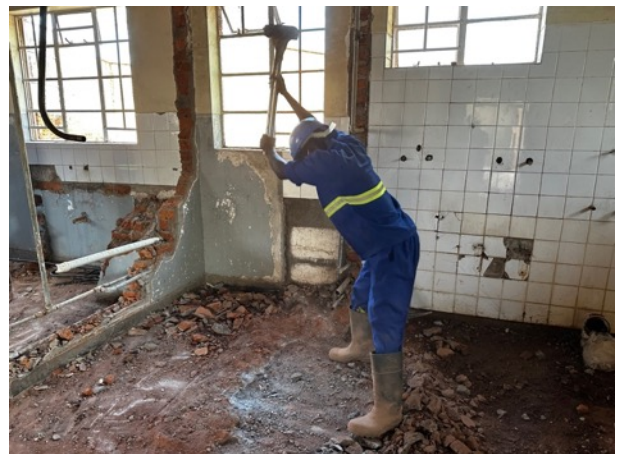
Demolition of old sluice area.
