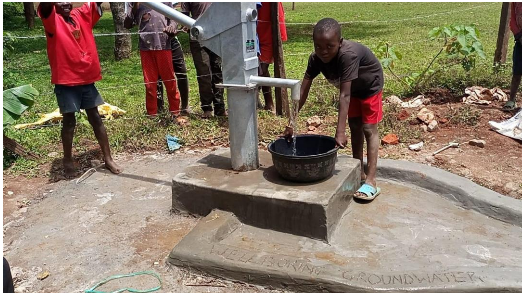
Pupils fetching water from the newly constructed well at Kisiombe Nakholo
