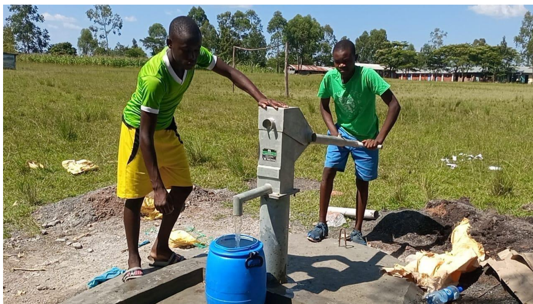
Pupils fetching water from the newly constructed well at Ataba Aburi
