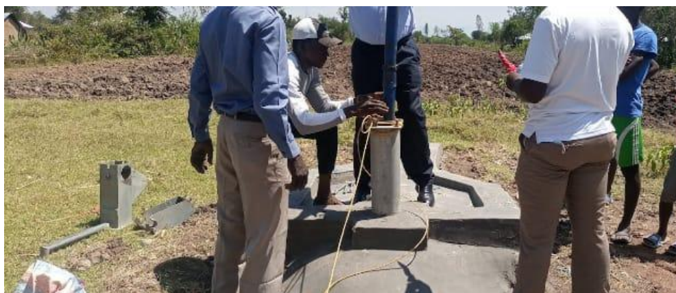
Pump installation at the newly constructed well
