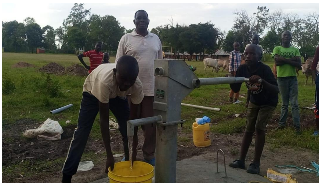
Pupils fetching water from the newly constructed well at Akibui
