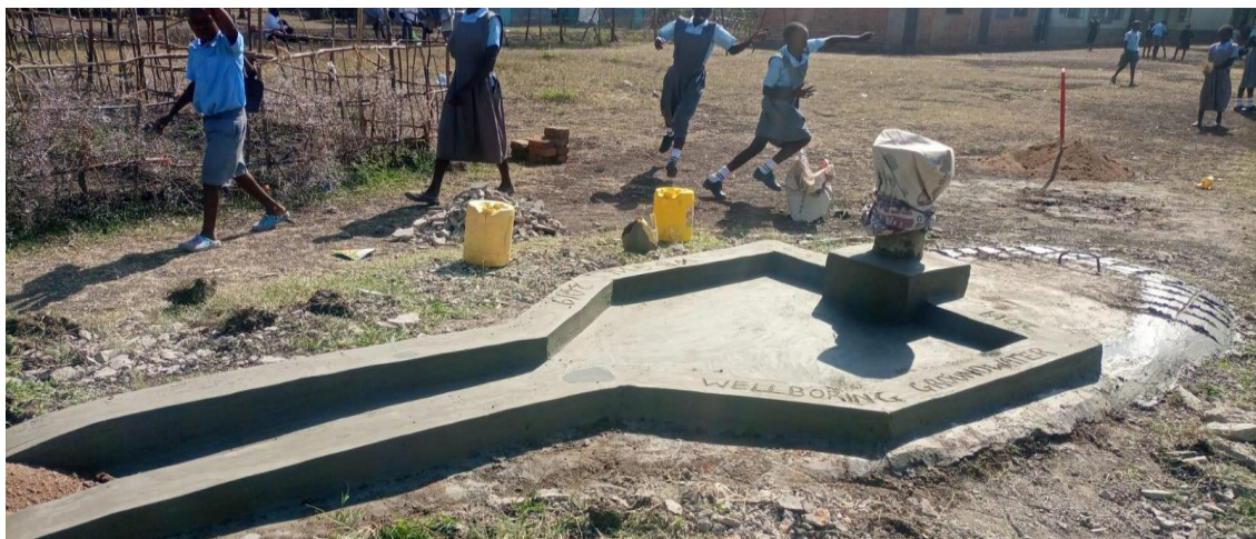
Pad construction at Kawalun Chakol Primary
