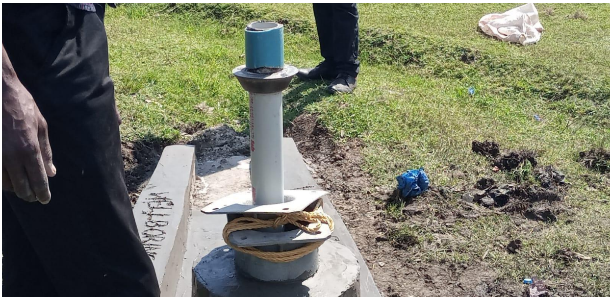
Pump installation at the newly constructed well
