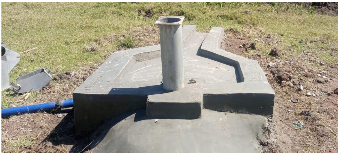
Pad construction at Kisiombe Nakholo Primary
