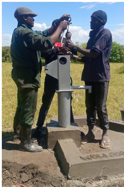
Pump installation at the newly constructed well
